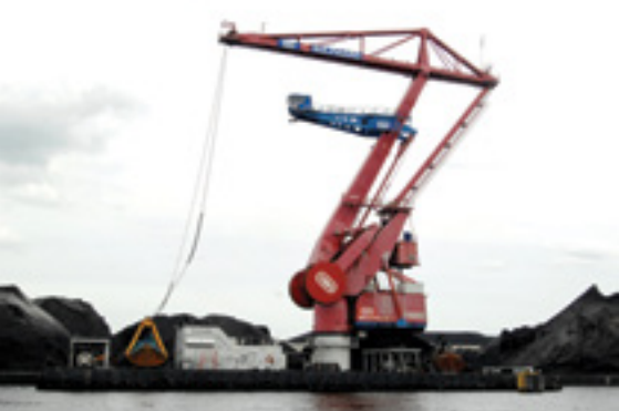
Figure 4.17 Typical grab crane. Courtesy of Pim Stouten
