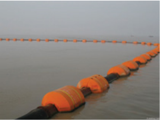
Figure 3.81 HDPE pipe with buoyancy elements
